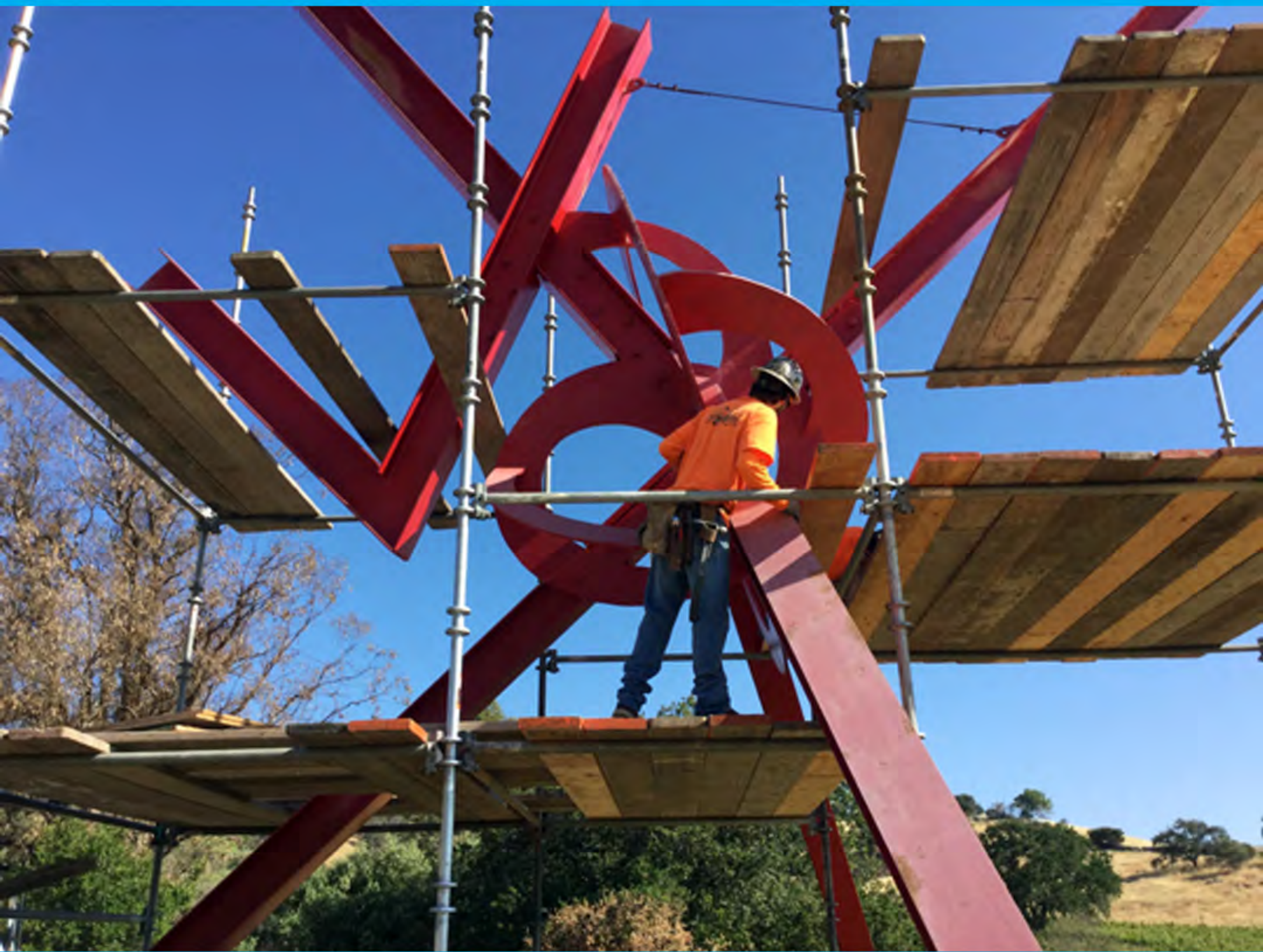
Scaffolding being installed around Mark di Suvero's For Veronica (1987) by Extreme Scaffolding
